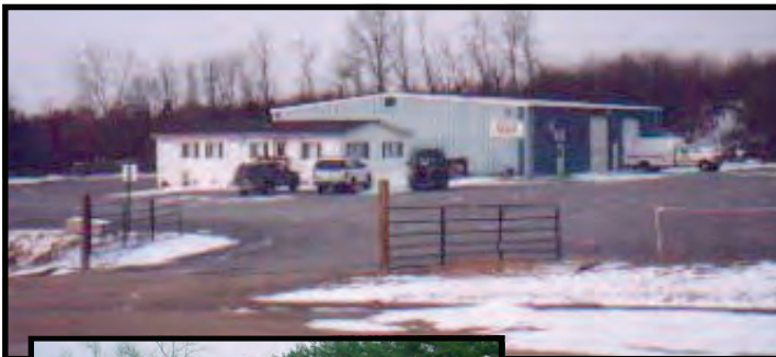
Cranberry Facility and yard, 2001
